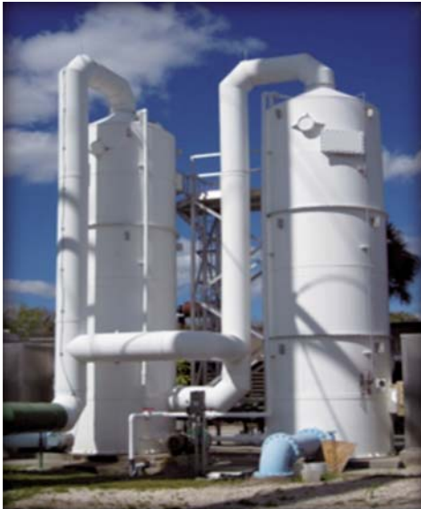
Figure 2. Forced Draft Aerators
